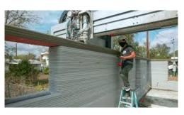
automatic troweling tool that flattens the 3D-printed layers and covers the grooves at the interlayer interfaces, resulting in a smooth concrete surface. The computer-controlled device is a gantry-style 3D printer with robot arms. (See: REFERENCES – ICF & 3D Printed Homes)
