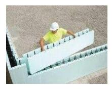
The many advantages of using ICF construction includes: energy-saving, dampen outside noises, and are fire resistant for up to 4 hours. Additionally, because EPS and concrete do not contain materials that promote organic growth, ICFs are resistant to mold and mildew growth and the resulting degradation that often occurs in wood frame structures. Independent third-party tests have verified EPS insulation used in ICF construction will not support mold growth (See "Moisture and ICFs: The Fact's).
